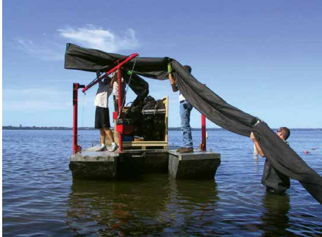
Figure 4. Boom wall being unloaded from a barge, June 2012 (photo: R. Lathrop, WDNR).
