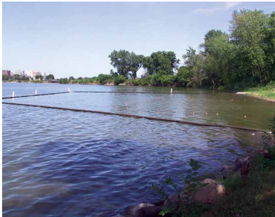
Figure 8. Deflector boom system deployed at Bernie’s Beach, June-August 2010-2011 (photo: R. Lathrop, WDNR).
