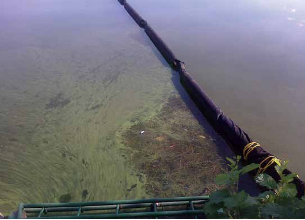
Figure 9. Algae scum and other floating debris trapped outside the sidewall boom at Bernie's Beach, July 2010 (photo: G. Steinhorst, City of Madison Engineering Dept.).
