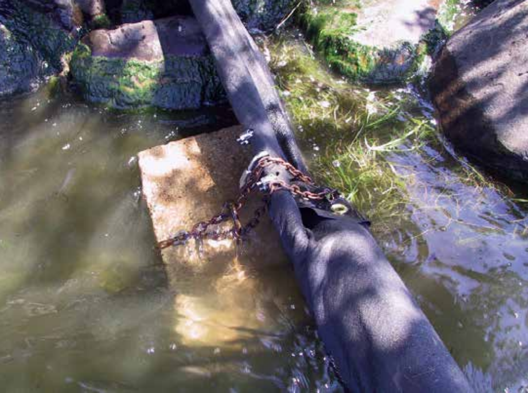
Figure 5. Concrete block and chain used to prevent boom wall from being lifted out of lake at shoreline (photo: R. Lathrop, WDNR).
