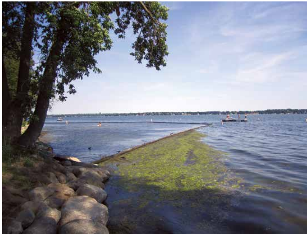
Figure 6. Photo showing the deflector boom system preventing algal scums and other floating debris from entering the enclosed swimming area at B.B. Clarke Beach, June 2012 (photo: C. Betz).
